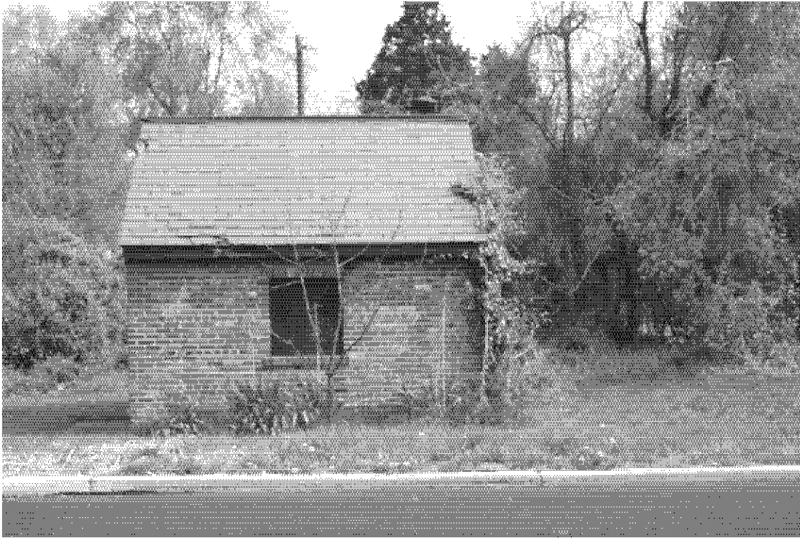
Figure 94: Oil storage house, Fort Hunt Park, 2004.
