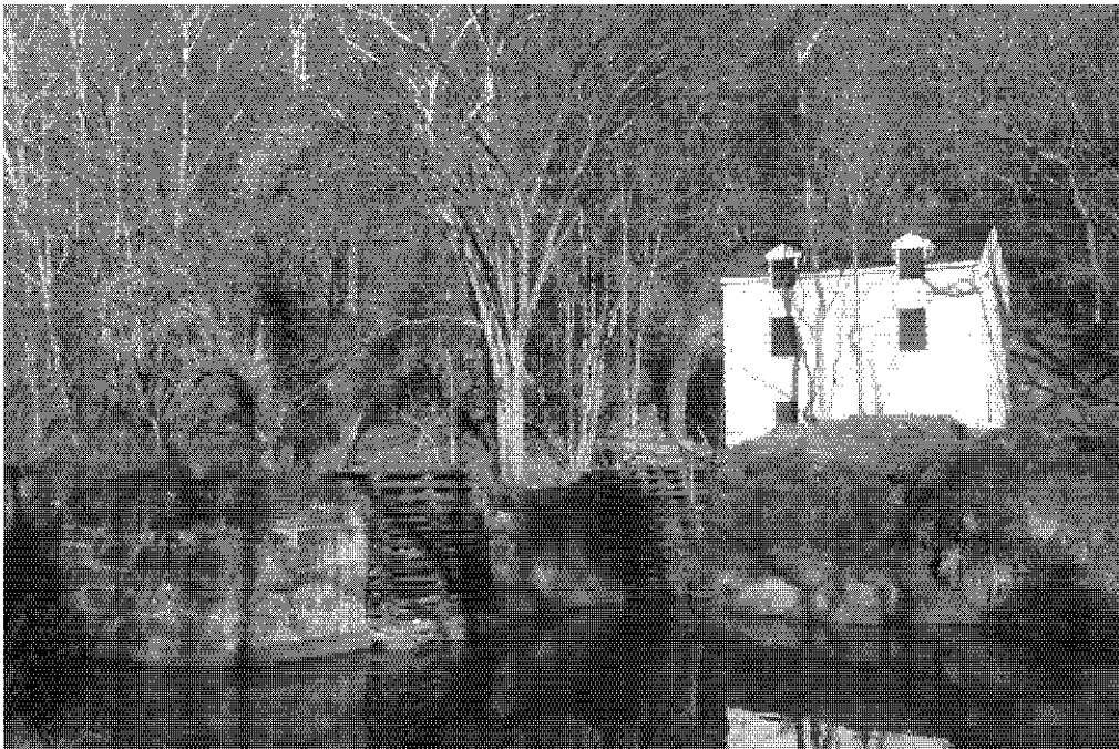
Figure 72: Restored lock house and bypass flume at Lock 15 along the C&O Canal, 2004.
