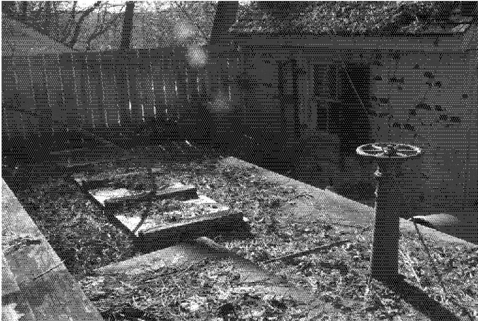
Figure 76: Up-hill side of water filtration plant building with extant mechanical equipment, 2004.
