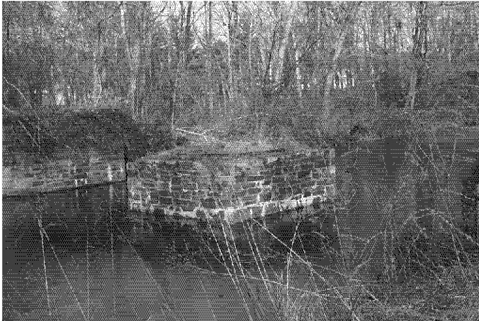
Figure 74: Footings of the swing bridge constructed near Camp NP-1-MD, 2002.
