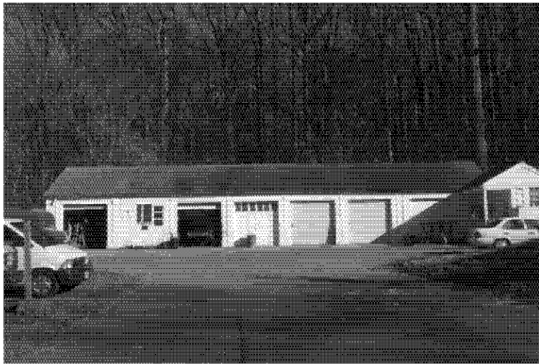
Figure 78: "Engineer's Garage," utility area above the Great Falls visitors area, C&O Canal, 2004.
