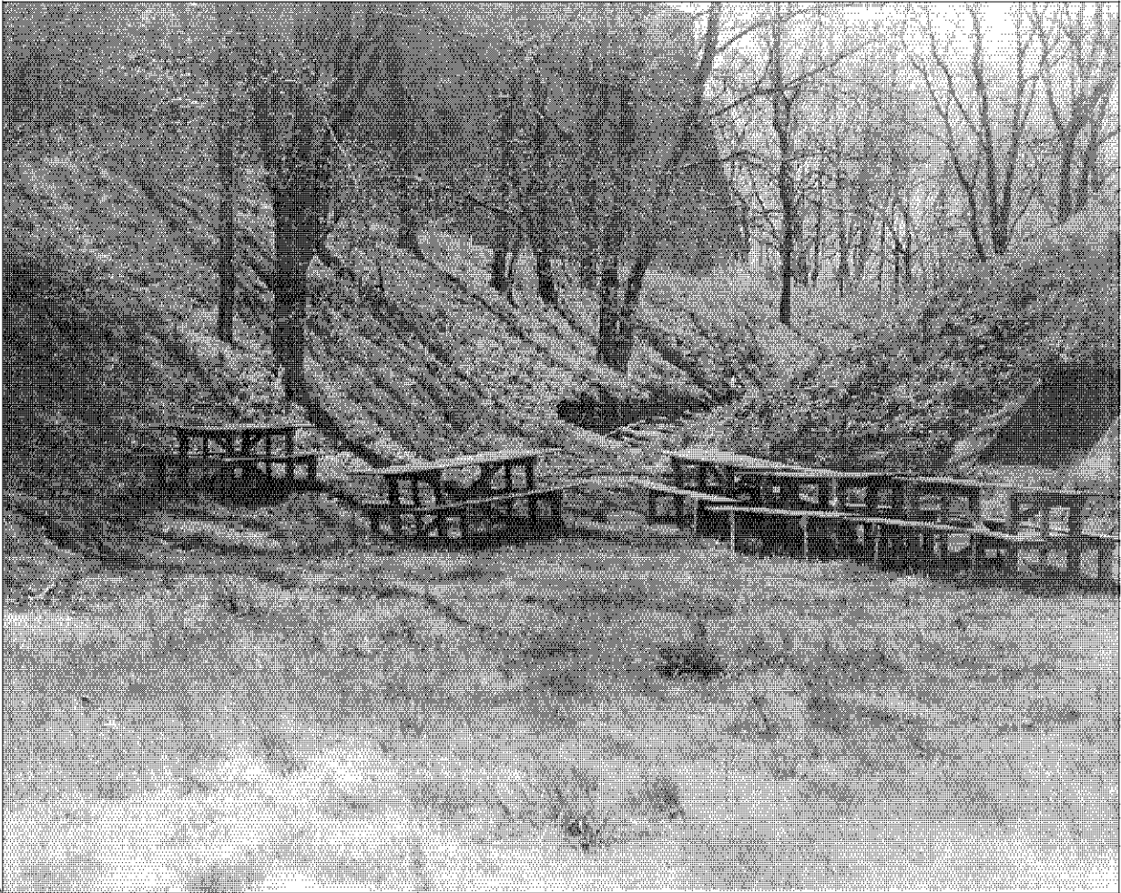
Figure 63: "Picnic Ground Development - Fort Washington," c. 1941. Source: RG 79-CCC, Still Picture Branch, NARA.
